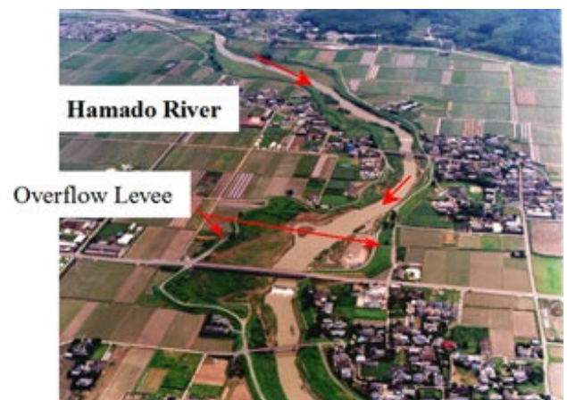
Figure 3 Kutsuwa Domo(Overflow Levee ) for Flood Protection/Mitigation at Shimada Dist., Hamado River (Field Study)
